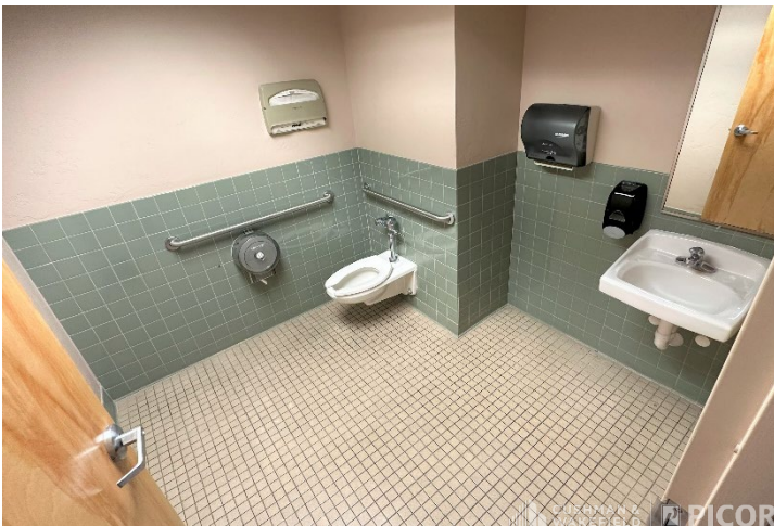
ADA Compliant Restrooms
