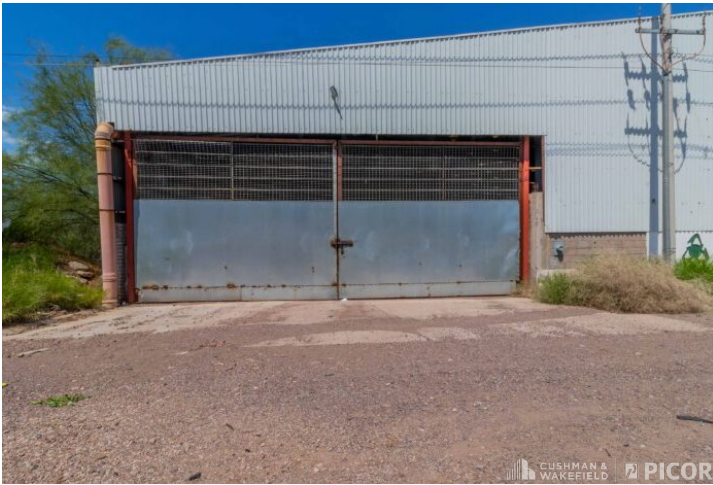
Secured Loading Area
